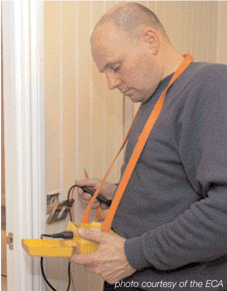
Testing Electrical Work
